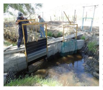
The other headgate was installed at the mouth of the West Ditch which feeds water to two irrigation canals where there was currently no water control structure. Having a headgate on the West Ditch will allow this ditch to be closed when outside of irrigation season, sending more water down the drain to Pahranagat National Wildlife Refuge.
